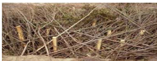
live branches installed in crisscross configuration.
